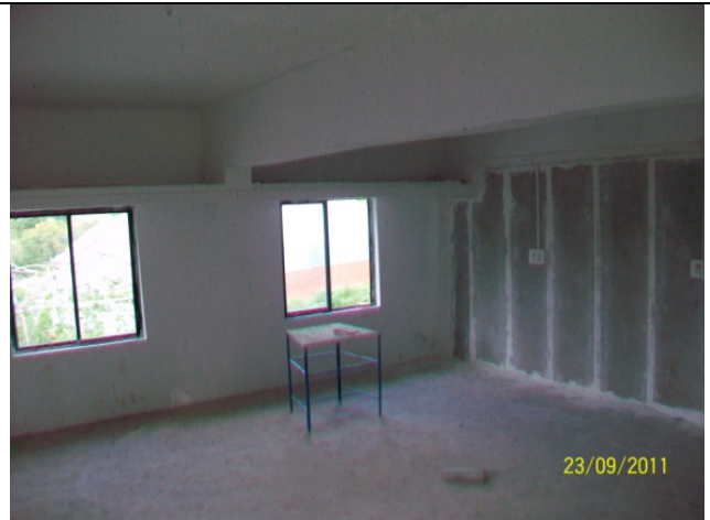
Partition in the basement
