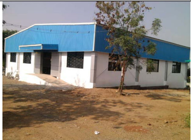
GKN finishing School building
